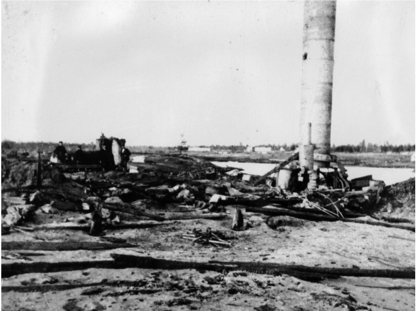
Men surveying what remains of a factory next to the Peshtigo River.
